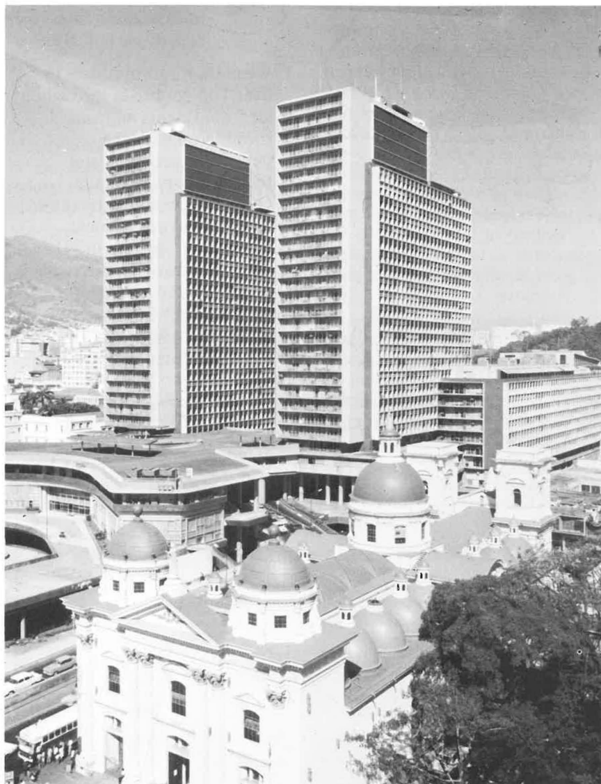
Twin 32-storey Simon Bolivar Centre, located in the capital city Caracas
